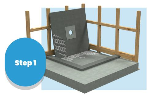
1. Apply cement based tile adhesive on the base and the floor using 10mm notched trowel to glue down the underlay to the floor.
