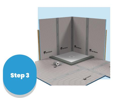
3. Apply a bead of polyurethane on the stainless-steel plate and plumber's glue to the drainpipe. Then fix the drainage flange in position and apply a bead of polyurethane to the outside of the flange. After the shower tray system is in place, install the wall sheeting, Seal joints with MARMOX sealing tape and cover all washers with MS Polymer.
