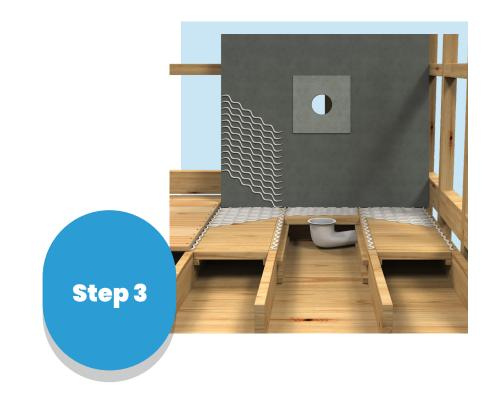
3. Use a polyurethane adhesive (non-solvent based) to glue down the underlay to the floor.
