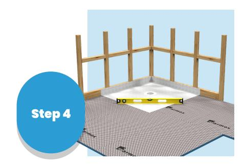
4. Place the underlay in position, apply downward pressure on the underlay and check for level.
